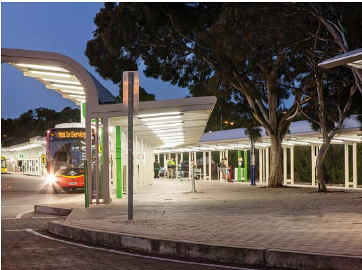
TEA TREE PLAZA BUS INTERCHANGE, AUSTRALIA
