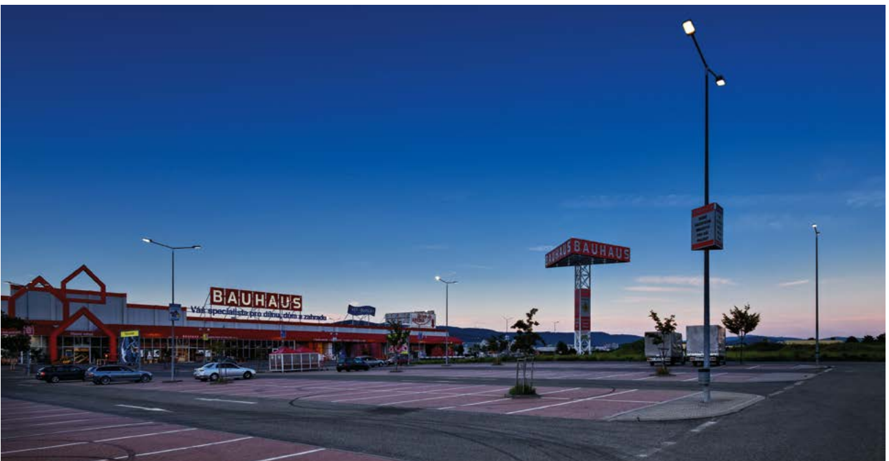
BAUHAUS CAR PARK, CZECH REPUBLIC
