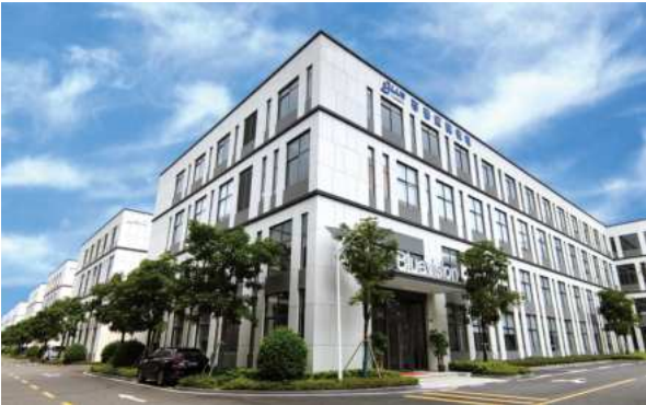
BLUEVISION (JIANGMEN) OPTOELECTRONICS CO., LTD (Factory) Building 2, Liandong U valley, No.32 Hexiang middle road, Hecheng Town, Heshan, Jiangmen City, Guangdong Province, China
